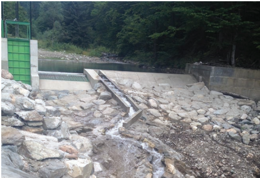
Photo1. Intake water and fish pass (SHPP Taia)
